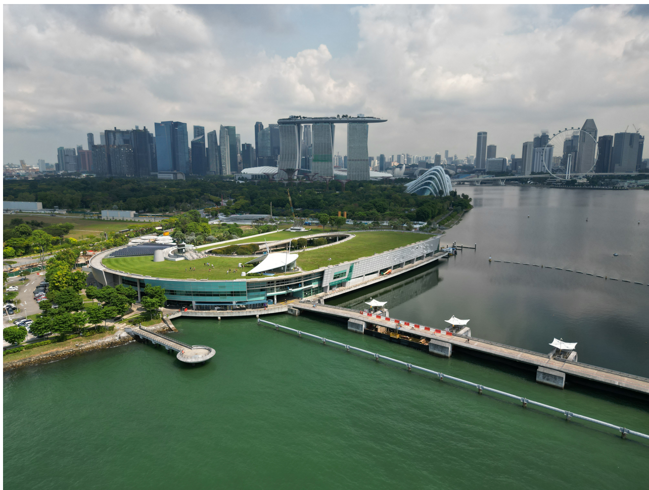
Figure 2. Marina Bay Barrage CloseUp, Singapour 2024, Crédits Bob Tan.
